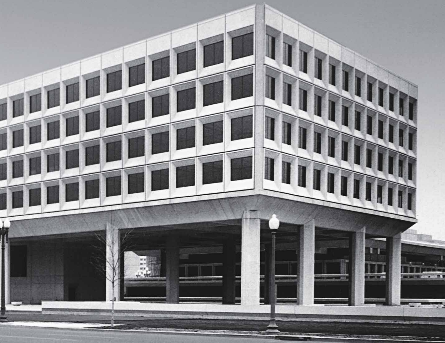
JAMES FORRESTAL FEDERAL BUILDING, WASHINGTON, DC | CURTIS & DAVIS | 1969
