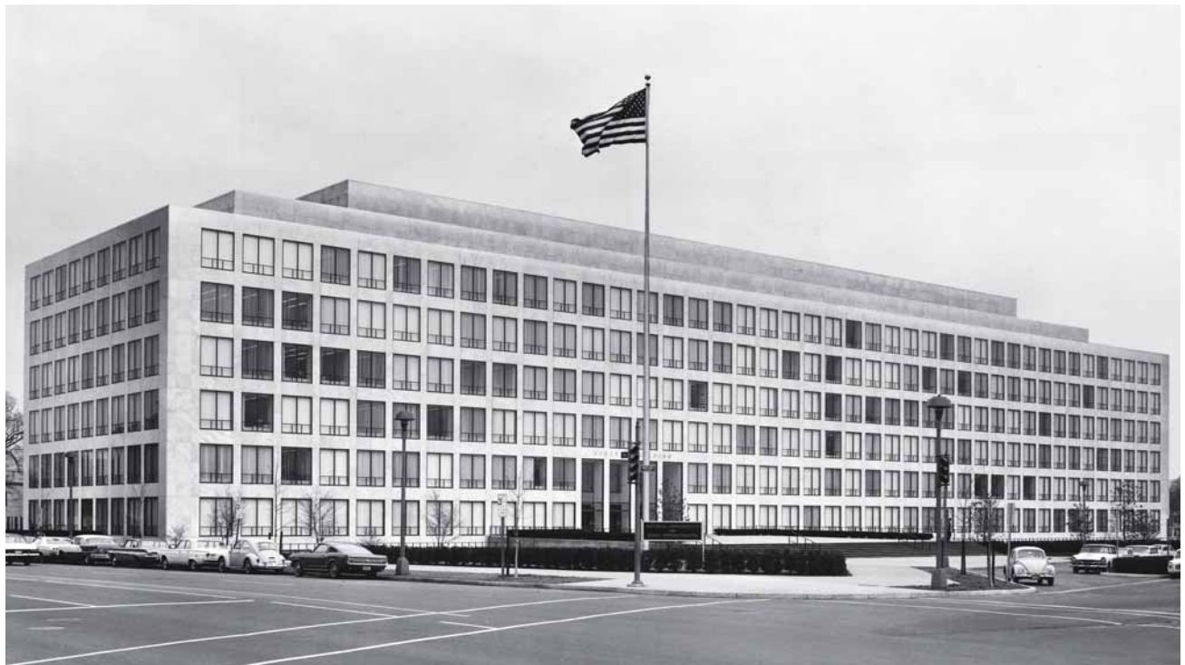
FEDERAL OFFICE BUILDING 10B, U.S. DEPARTMENT OF TRANSPORTATION, FEDERAL AVIATION ADMINISTRATION, WASHINGTON, DC | HOLABIRD, ROOT & BURGEE AND CARROLL, GRISDALE & VAN ALLEN | 1963
