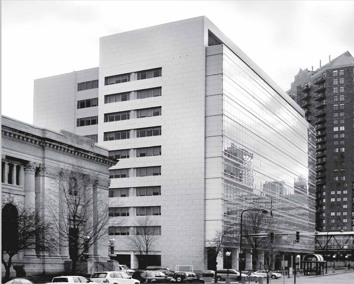
FEDERAL BUILDING | DES MOINES, IOWA | WETHERELL HARRISON WAGNER AND MCKLEEVEN | 1967-68 | NEUMANN BROTHERS | 2002
