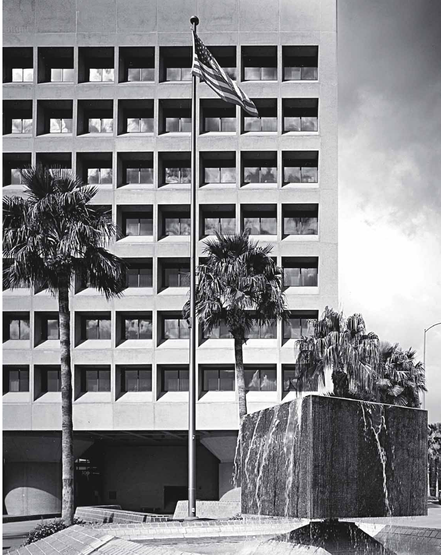
FEDERAL BUILDING, TUCSON, ARIZONA | CAIN, NELSON, WARES, COOK & ASSOCIATES | 1974
